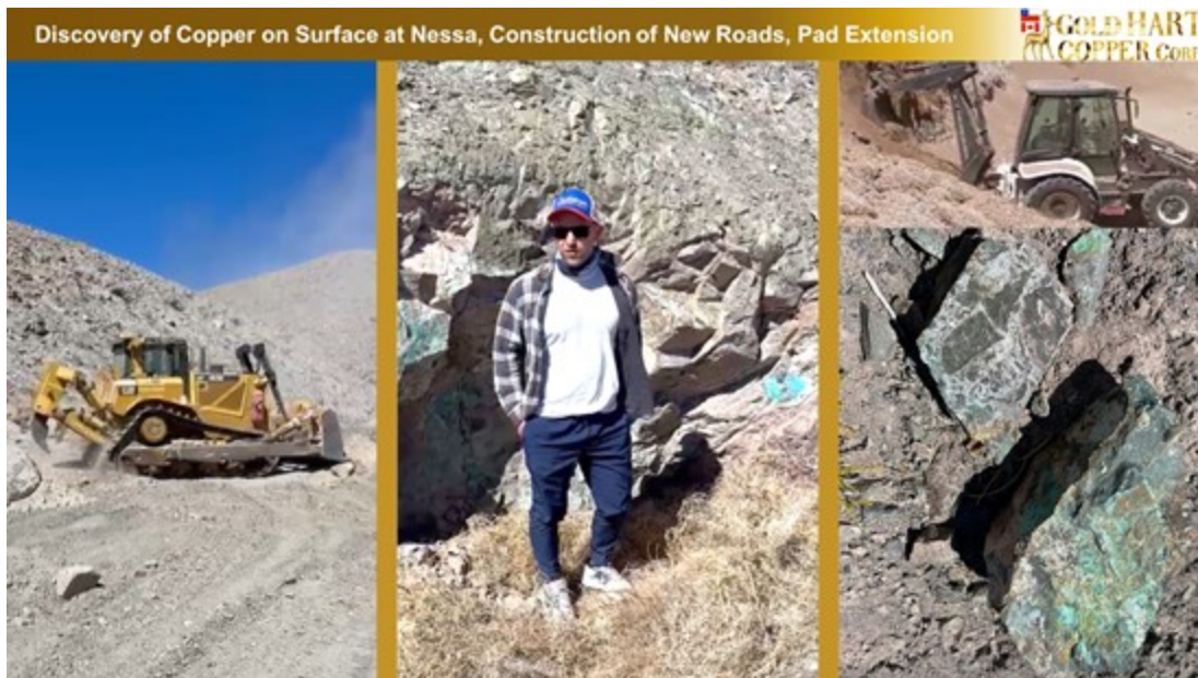
Copper on Surface Nessa - New Pits - Road Construction
