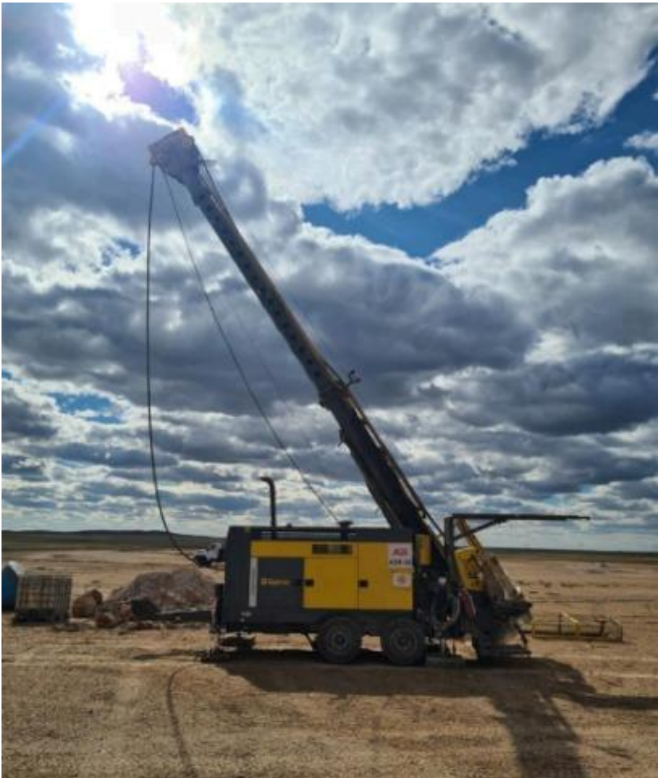
Figure 39: AQS Christensen 140 drill-rig
