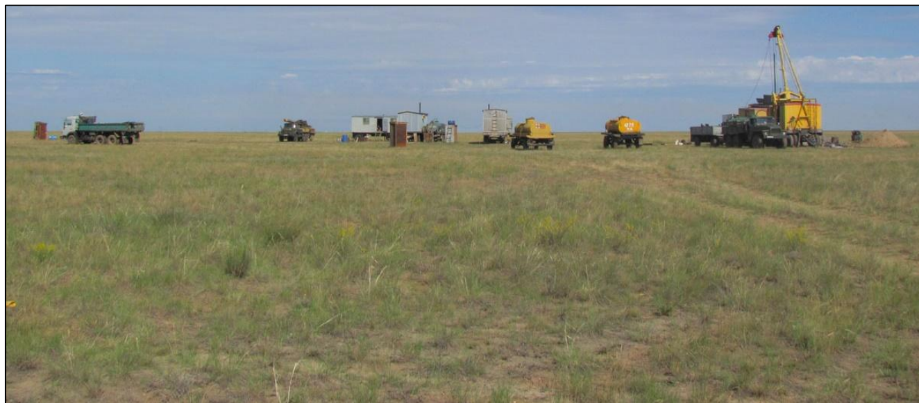
Figure 4. Drilling at the Elemes Project
