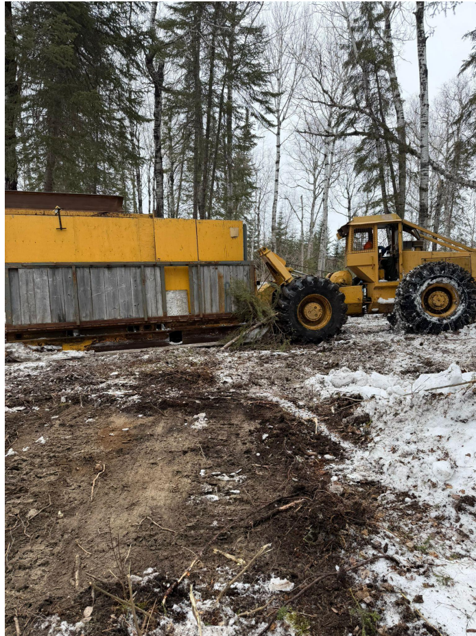
Image 2: Drill and Skidder on Location
