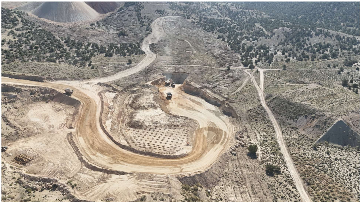
Figure 3 – Heap Leach Pad advancement as at June 16, 2026
