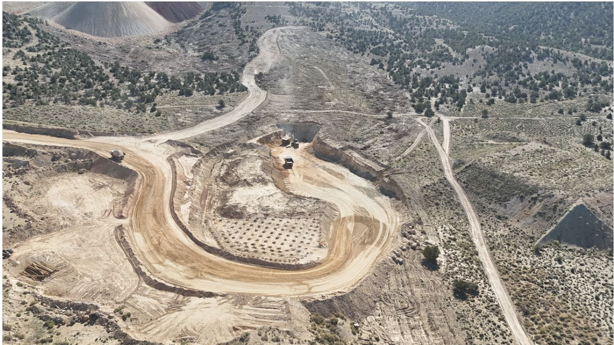
Figure 3 – Heap Leach Pad advancement as at June 16, 2026
