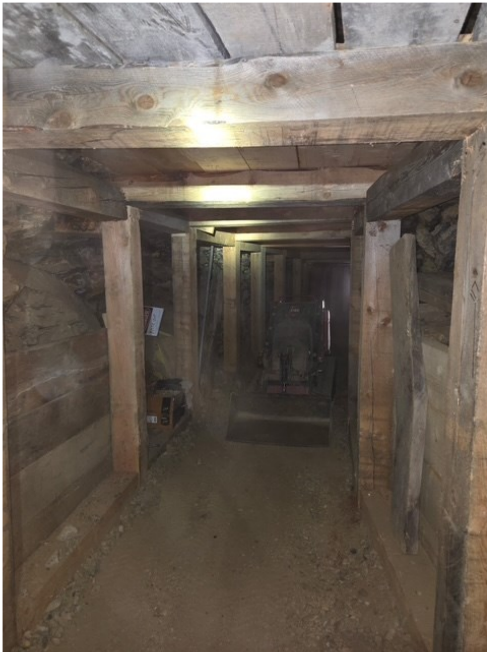
Zero Level - Rehabbing of the access drift
