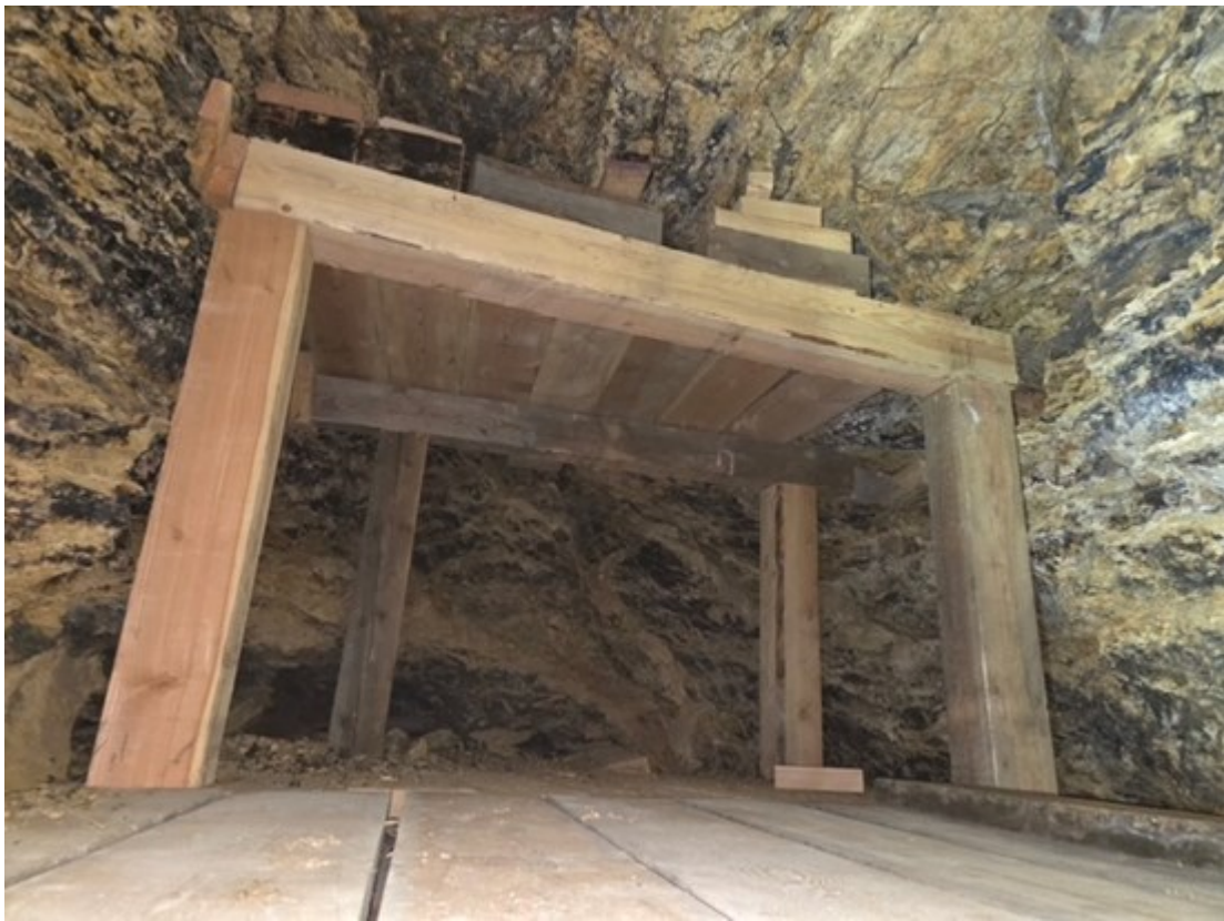
Zero Level Access Drift - Additional Support Installed
