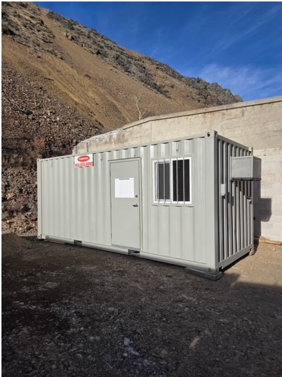
Base of Canyon - New Office Container
