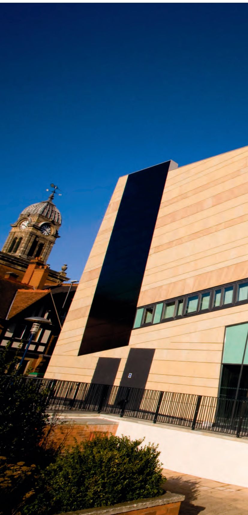
Stanton Moor Sandstone Cladding, Derby
