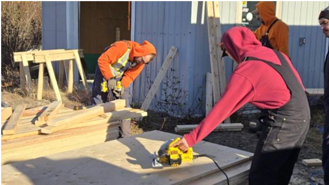
Figure 2: Brandon Sainsbury and Saga Technicians building core facility in Cartwright
