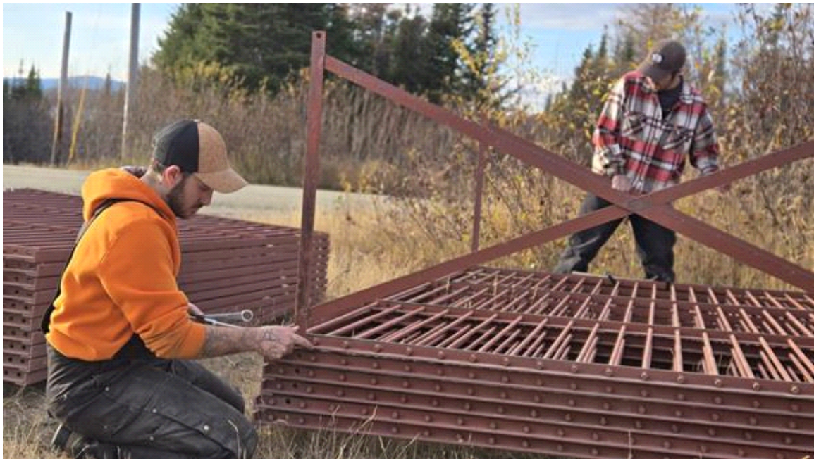
Figure 3: Saga's team from Cartwright preparing the metal core racks on site.
