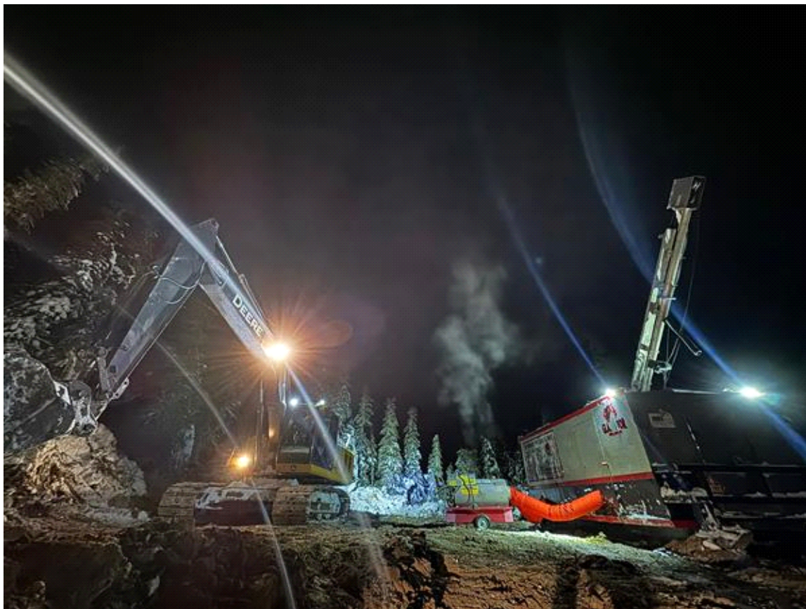
Figure 4: Gladiator Drilling's drill shack and 25-tonne excavator located on cross-section S8 commenced drilling hole R-0016 in Trapper South.
