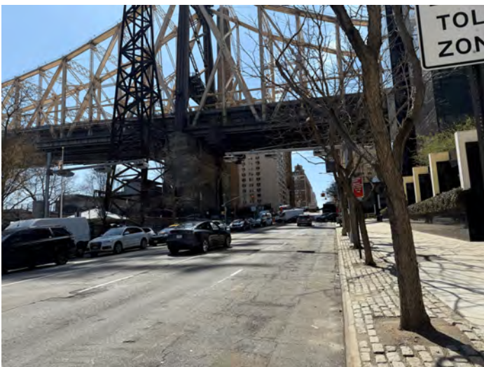
VIEW OF YORK AVENUE FACING SOUTH
