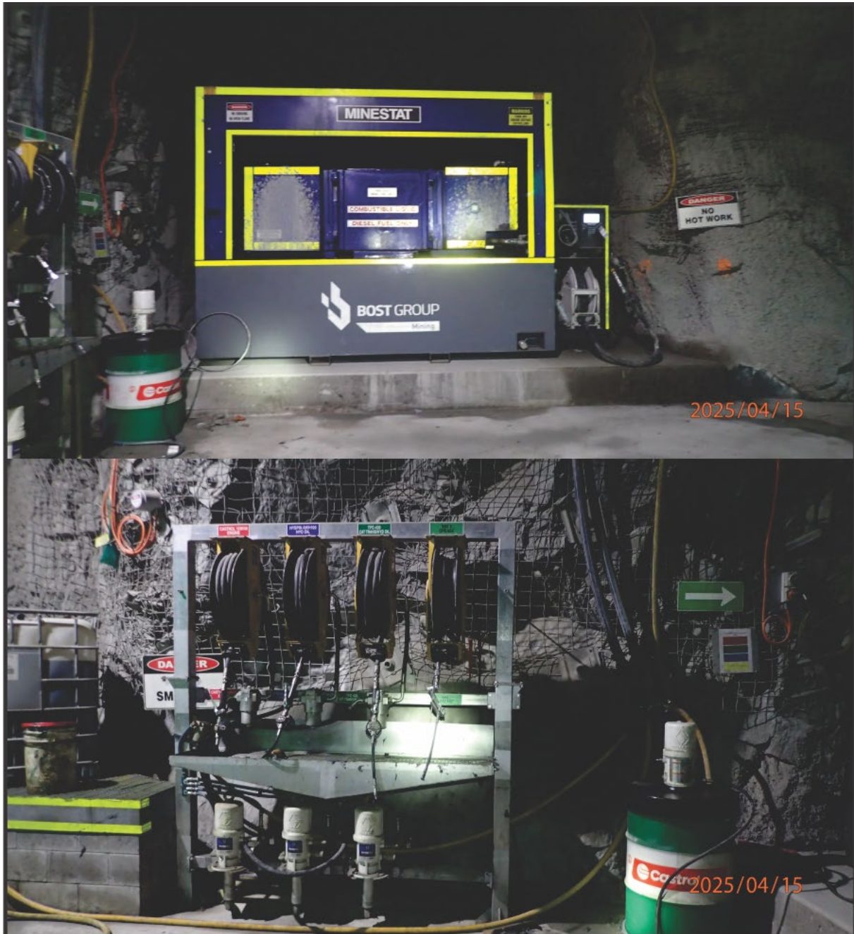
Figure 18-3: Roswell refuelling and lubrication facilities
