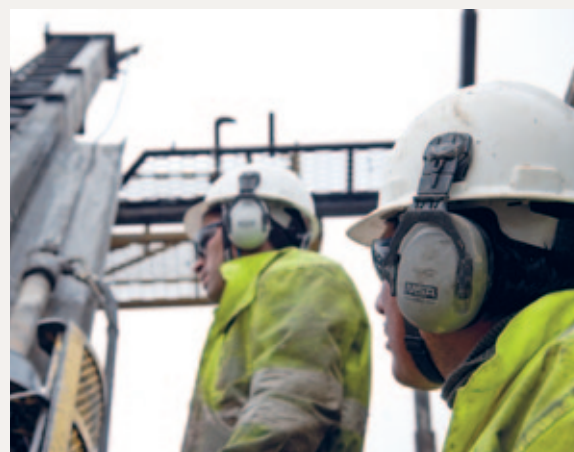
Employees operating a drill rig
