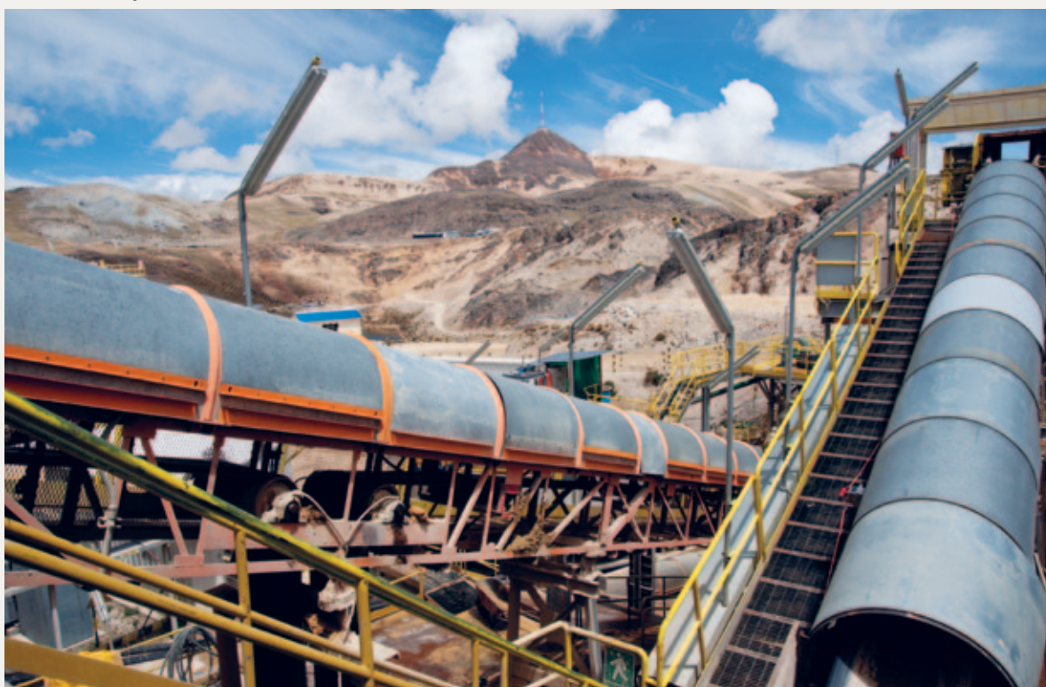
View of the Selene plant
