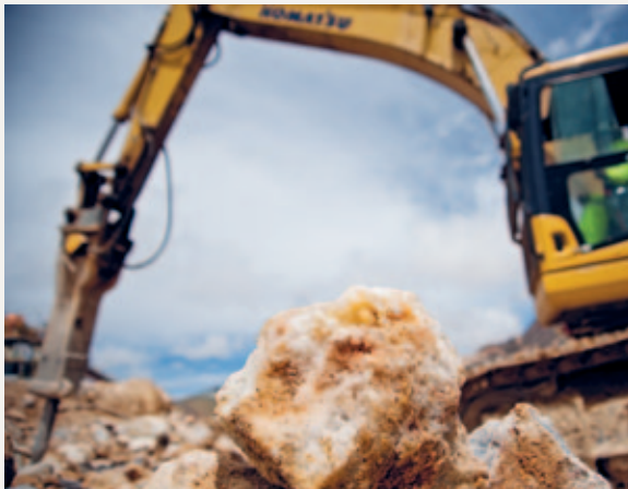
Work in progress at Pallancata
