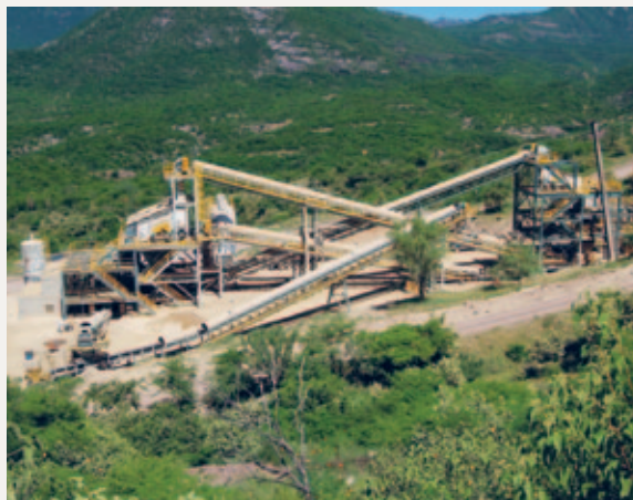
View of the plant at Moris
