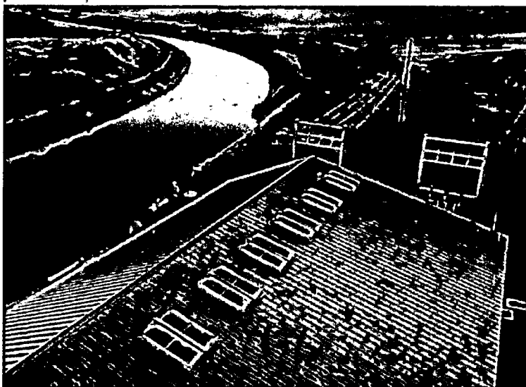
Pictured: The BILCO roof hatches provide natural daylight, allowing the facility to lower its energy usage costs.
