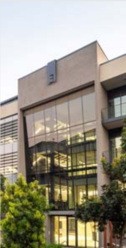
The Ingress – Building 3, Waterfall City
