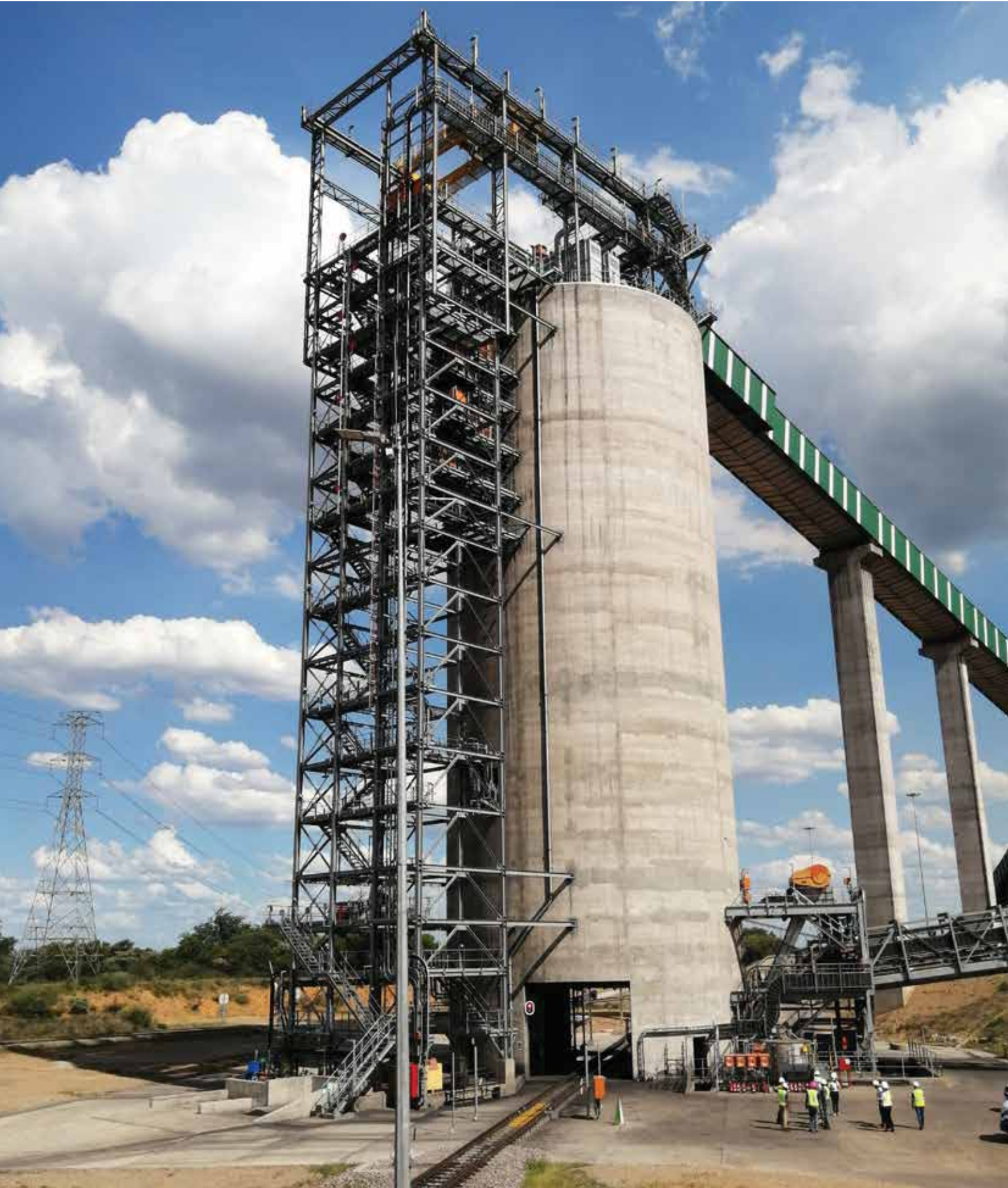
Load-out station at Grootegeluk
