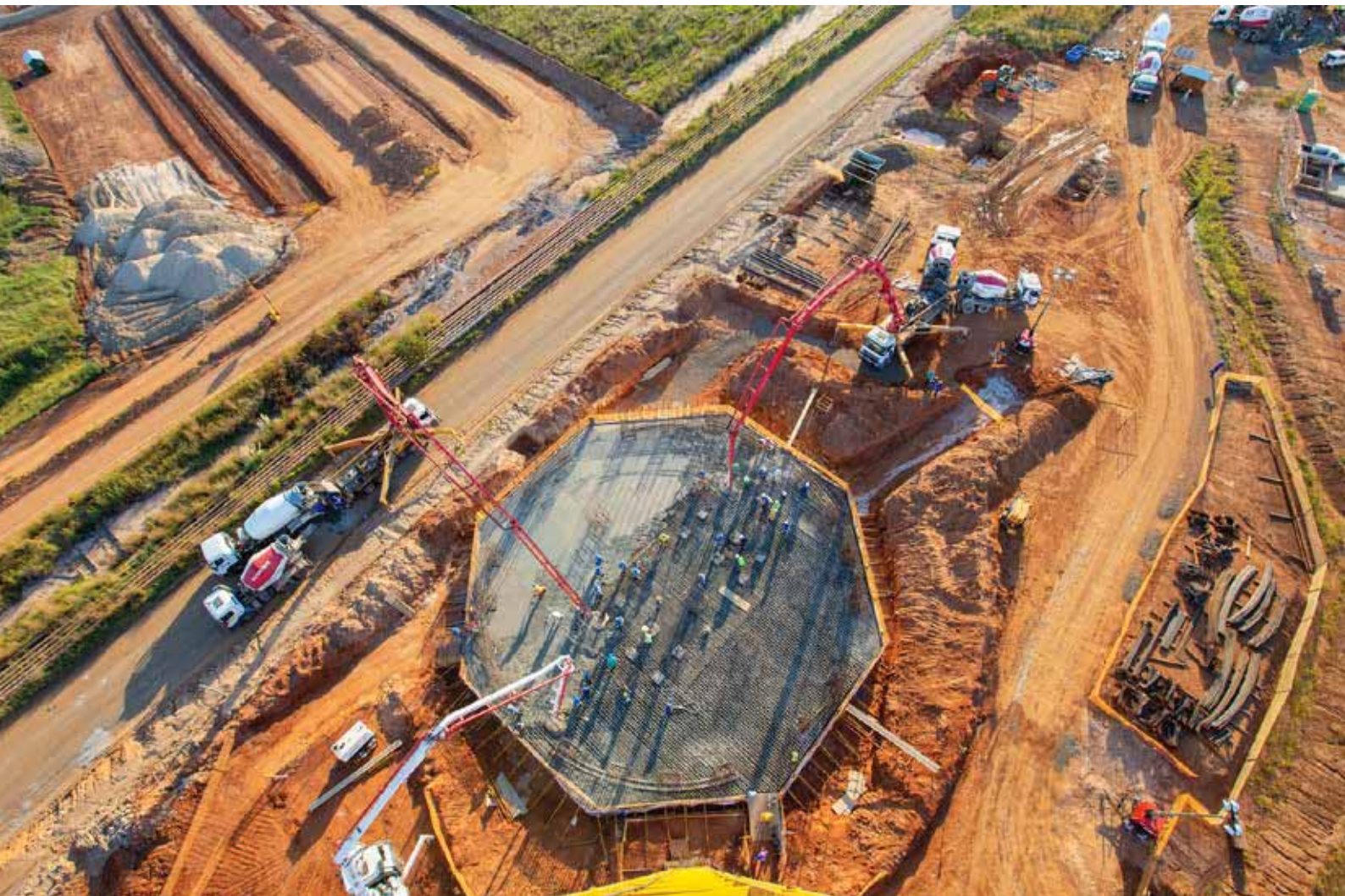
New shaft under construction at Matla Mine 1
