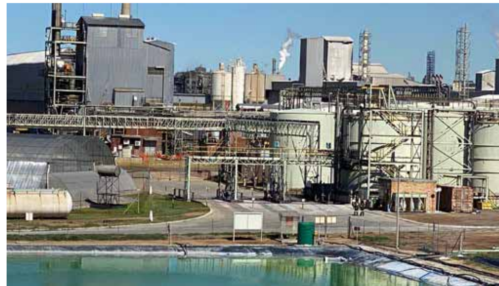
Emissions of nitrous oxide (NO x ) and nitrous oxide (N 2 O) are reduced to impact positively towards the improvement of the air quality of the Sasolburg area.
