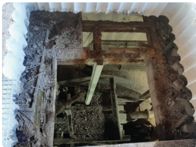
Photo 4: Hutchings Shaft Cement Slab Opened.
