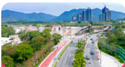
We improve local infrastructure by widening roads, building footbridges and cycling tracks in Sai Sha
