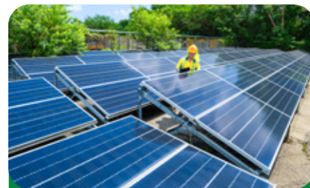
Solar farm at Sai Sha construction site
