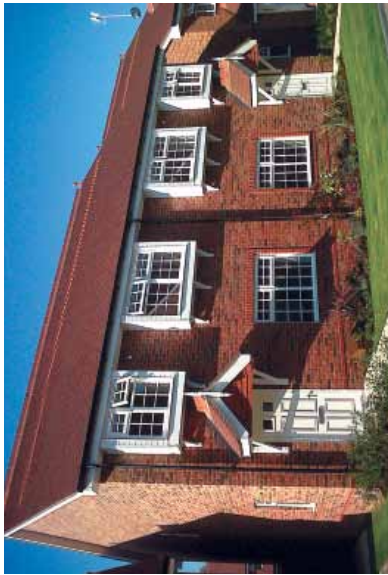
→ Completed homes at Woodland Chase, Croxley Green
