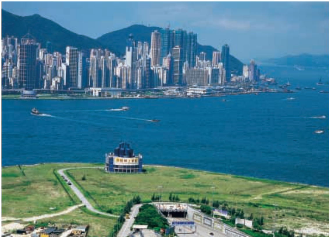
Entrance of Western Harbour Tunnel
