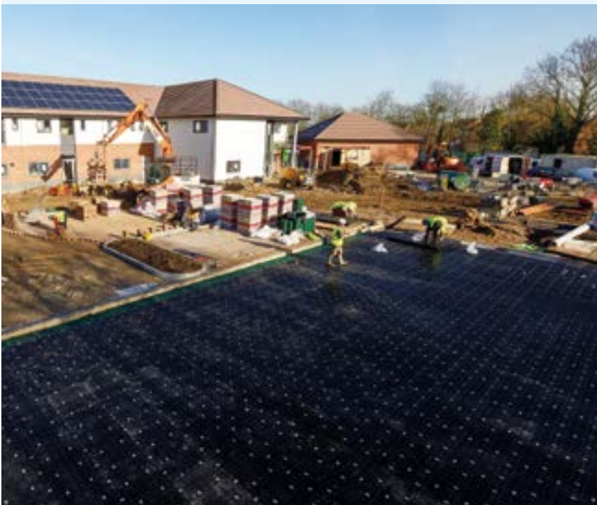
⌕ Permavoid cells being installed to prevent surface water flooding
