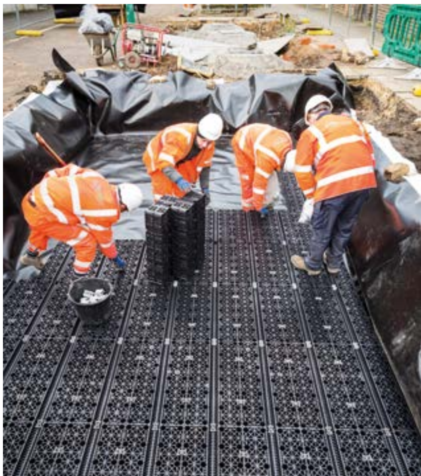
Ⓢ Permavoid being used for a rain garden installation, combining sustainable drainage with urban greening
