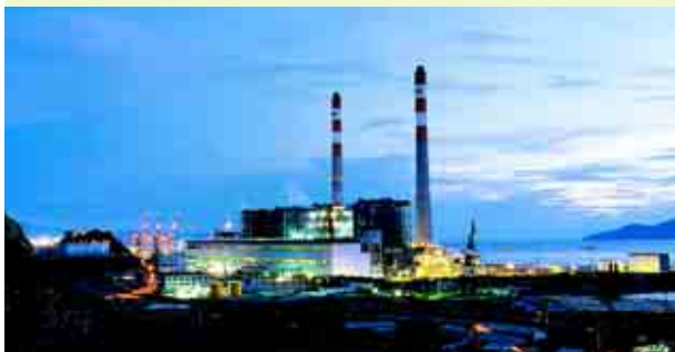
媽灣電廠 Mawan Power Plant
