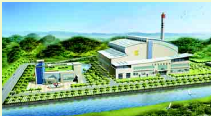
江陰垃圾焚燒發電廠 Jiangyin waste-to-energy plant
