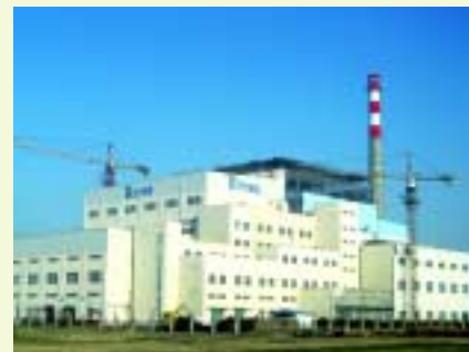
Yixing Waste-to-energy Plant 宜興垃圾焚燒發電廠
