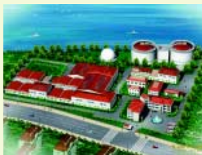
Qingdao Maidao Waste Water Treatment Plant 青島麥島污水處理廠
