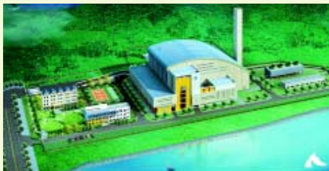
Jiangyin Waste-to-energy Plant 江陰垃圾焚燒發電廠
