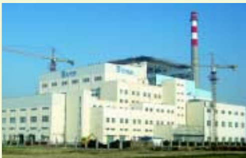
Yixing Waste-to-energy Plant 宜興垃圾焚燒發電廠
