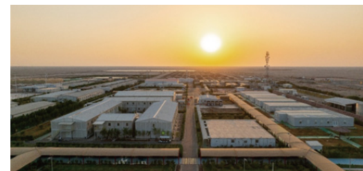
Overview of the Block 9 main camp
