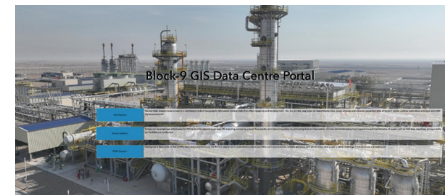
Block 9 GIS Data Center Portal
