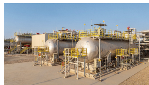
Overview of the Block 9 Central Processing Facility (CPF)
