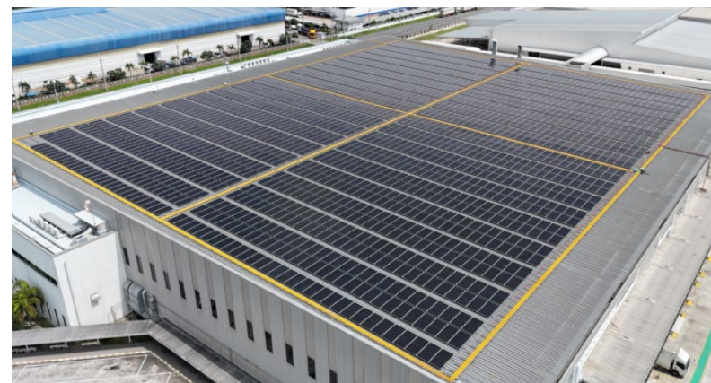
Rooftop Photovoltaic Project at Joyson Safety Systems Thailand Plant
