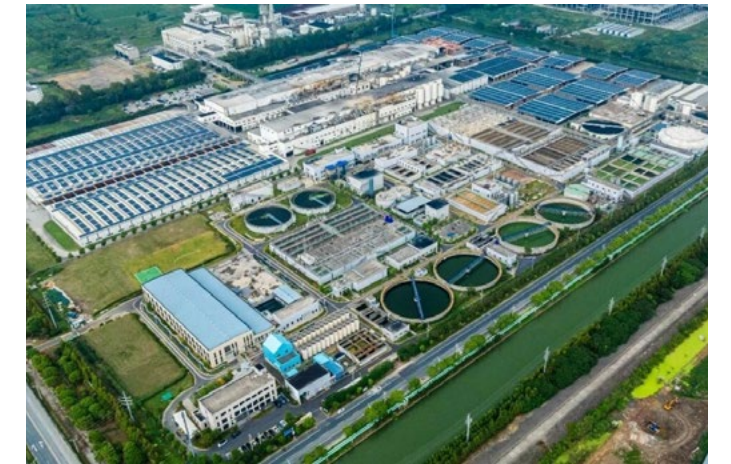
► Pinghu Wastewater Treatment Plant
