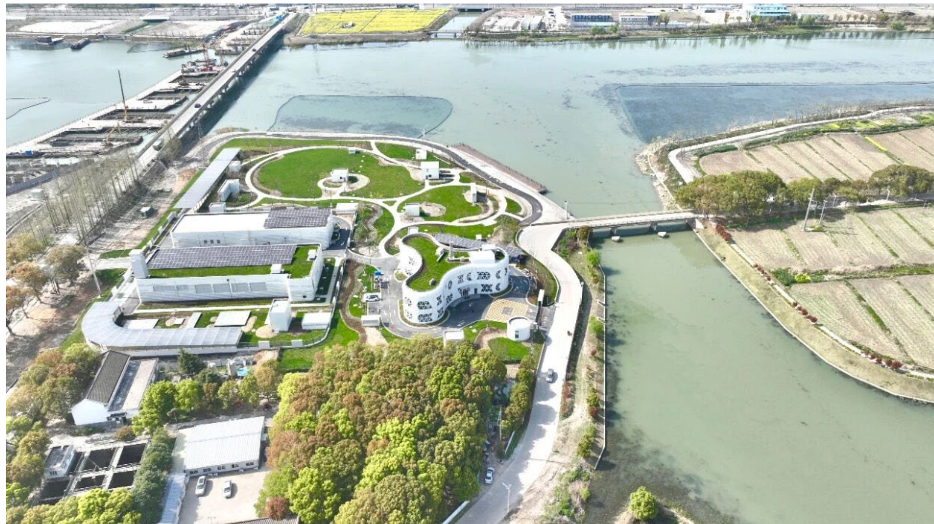
► Xicen Wastewater Treatment Plant Project
