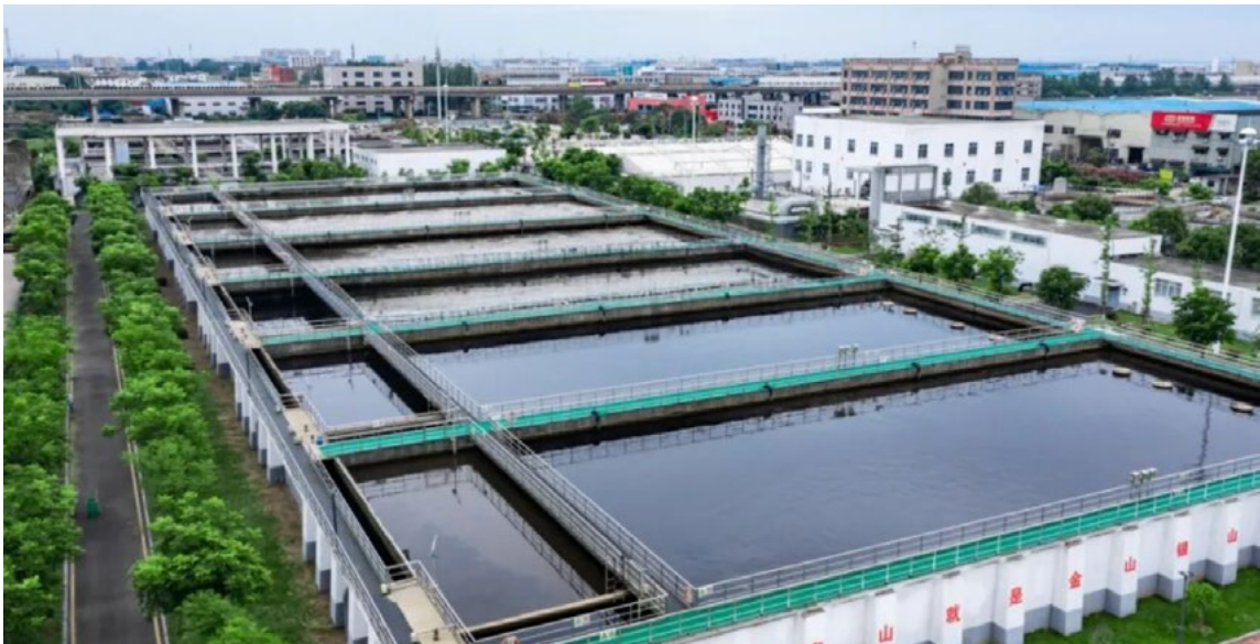
► Nanchang Xiaolan Wastewater Treatment Plant
