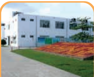
Danang City, Vietnam – First plant
