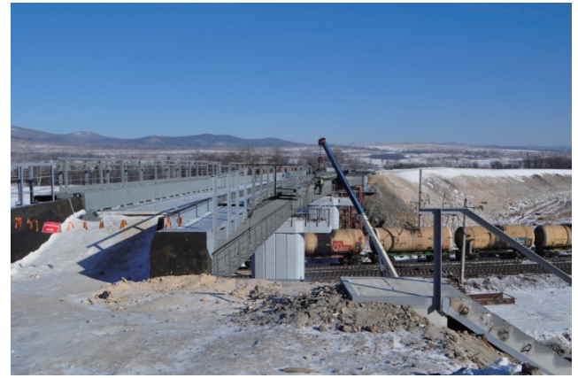
View across connected bridge
