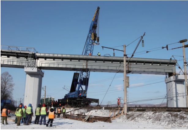
Central bridge section lowered into place
