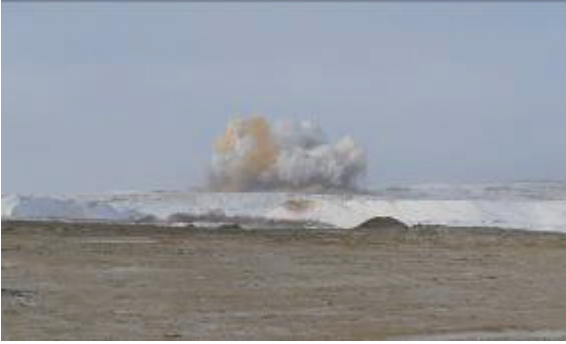
Blasting at Kimkan Mine
