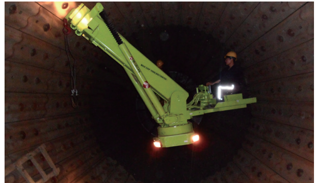
Ball mills lining being installed
