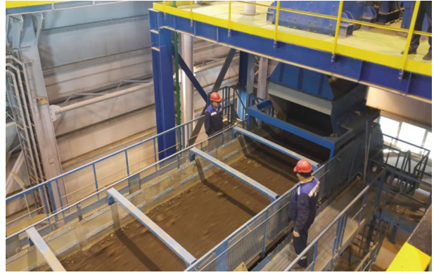
Conveyor belt at crushing and screening plant
