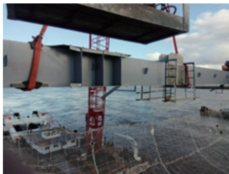
Construction of the Amur River Bridge in progress
