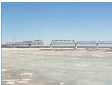
Amur River Bridge, due for completion in July 2019
