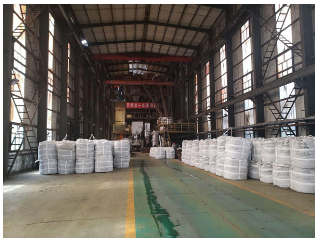
Vanadium JV-Smelting and packing facilities
