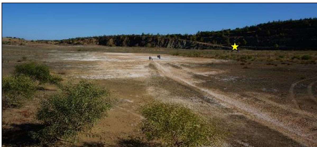
Figure 23 – Limni mine; backfilled (October 2017, Andrew Craig). Light coloured surface defines the seasonal pool extent with run-off running to the lower-right of the photo. See Figure 22 for view of open pit before infill; star for cross reference between the photos
