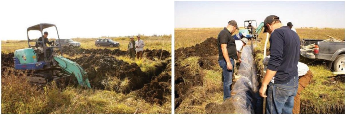
Figure 9-1: Trial In-situ leaching cell construction.
