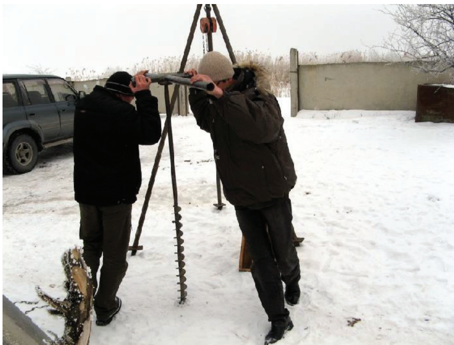
Figure 5-2: Manual Auger Drilling
