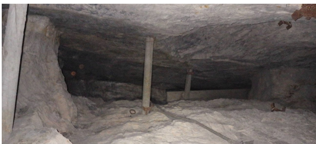
Photograph 13-1: Image of old stope, open and in reasonable condition
