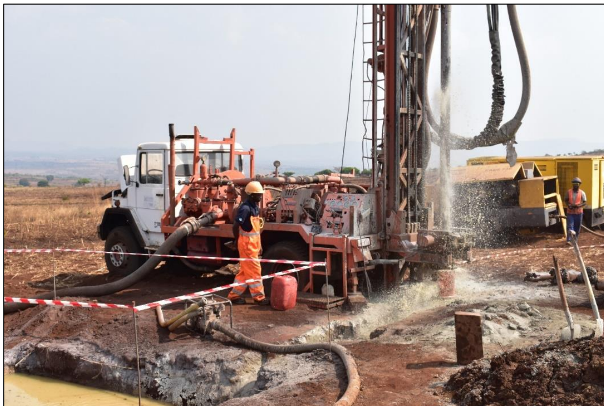
Figure 6-2: Water bore drilling – August 2019
