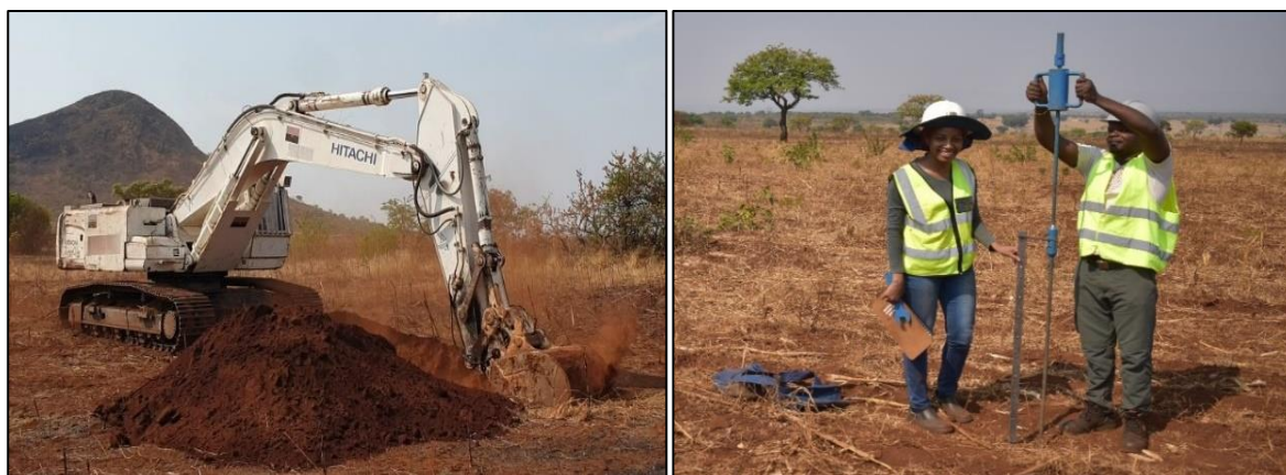
Figure 6-1: Geotechnical site investigations – August 2019
