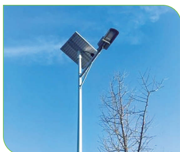
◇ Solar Street Light Retrofit
