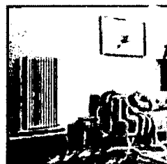
Decorative steel tubular and column radiators
