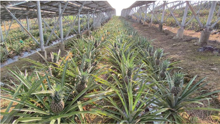
Pineapple cultivation at the Jiangmen Heshan Agricultural Photovoltaic Complementary Power Station (江門鶴山農光互補電站)
