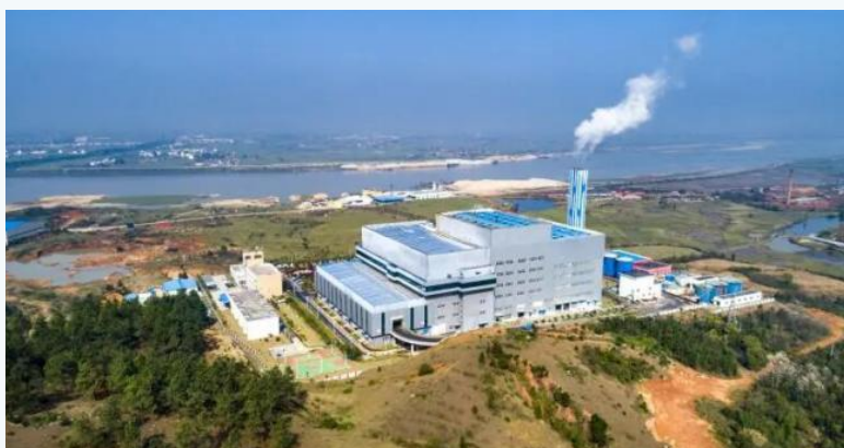
Nanchang Quanling Waste-to-Energy Plant
