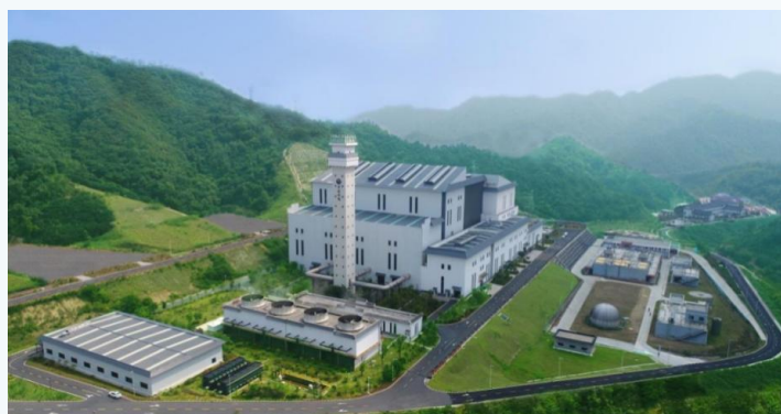
Panoramic View of the Huizhou Ecological Environment Park Waste-to-Energy Project
