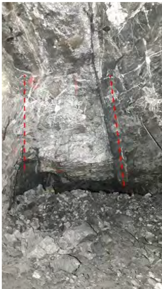
Figure 8-6 Waste Fill in C&F Mining Operation
