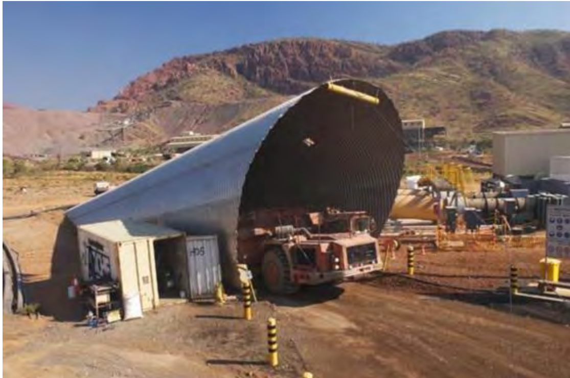
Figure 8-8 Buried Armco Portal
