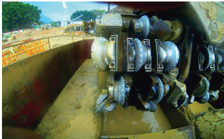
Roller cutters to diaphragm wall
