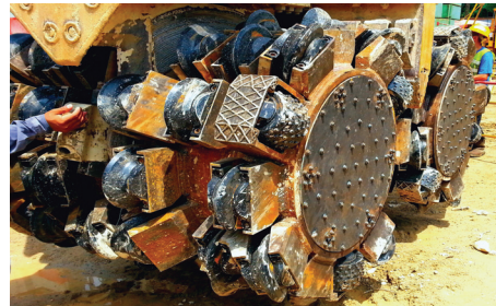
Roller cutters to diaphragm wall
