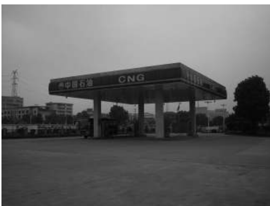
Vehicle Gas Filling Station at Deshan Gas Station
