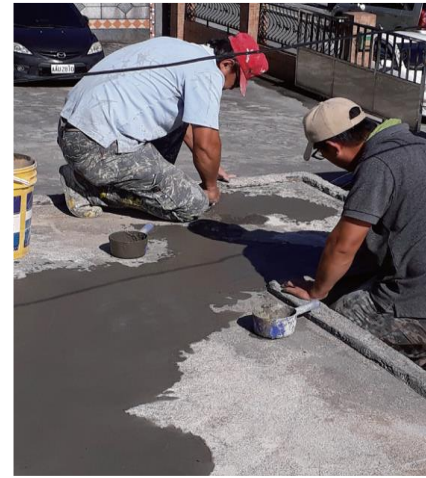
Free house repairing
