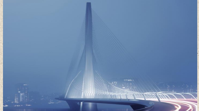
Danjiang Bridge is expected to open to traffic in 2024.
