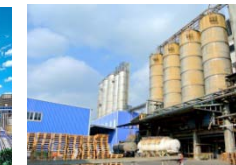
PA6 Polymerization Plant III , 2013
