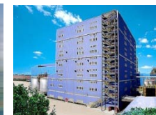
PA6 Polymerization Plant II , 2005
