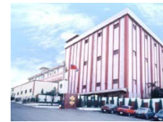
DTY Plant I 1969
