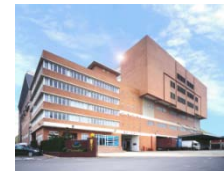
PA6 Spinning Plant I , 2000
