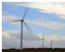
Wind Farm Power Plant
