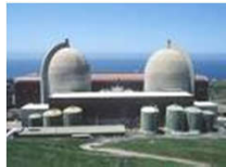
Nuclear Power Plant
