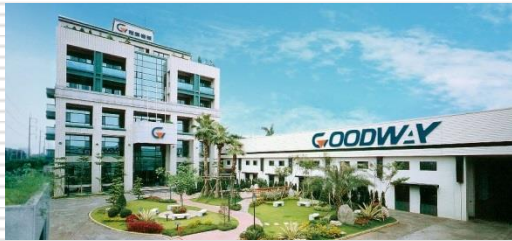
GOODWAY Headquarters / 18,600 m 2
