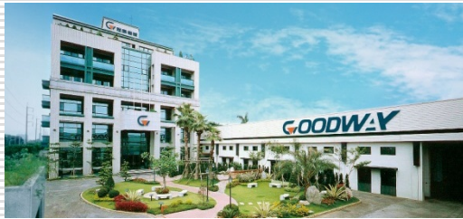
GOODWAY Headquarters / 18,600 m 2
