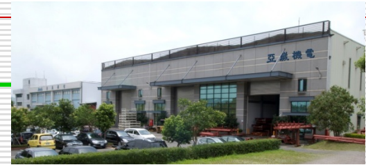
AWEA Headquarters / 26,000 m 2
